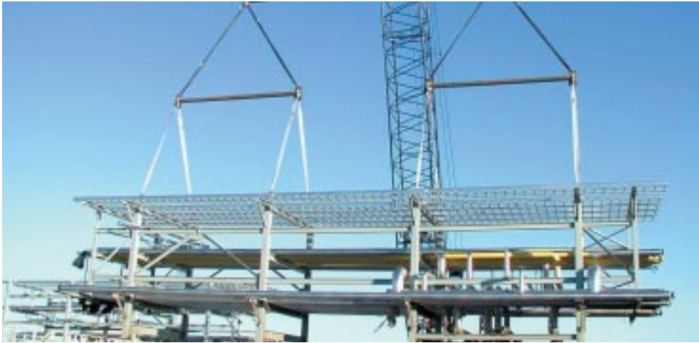
Triton: Module fabrication for the heavy oil sector
